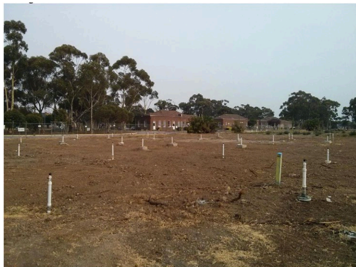
Organohalide respiring bacteria (ORB) bioaugmentation driven bioremediation rollout at Deer Park, Victoria.. Photos provided courtesy of Orica Australia and Golder Associates.
